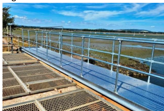
New bridge at Thorney Island – Sourced from sussexexpress.co.uk , 2025
