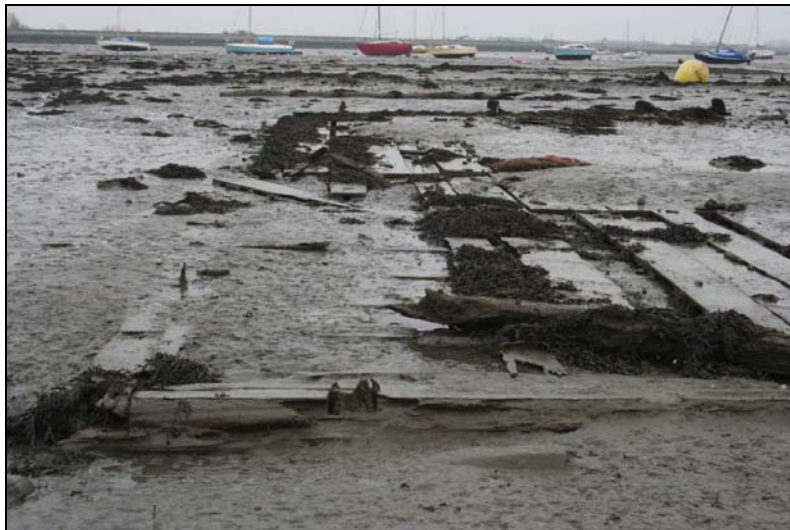
Figure 9: The partially exposed remains of the Ark.
