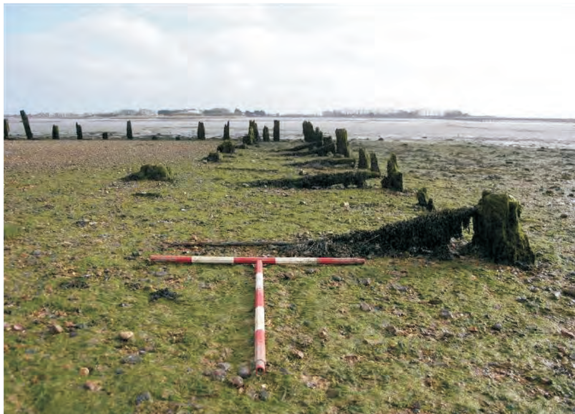
Fig 7 The wharf structure at Warblington, showing parallel piles with cross-bracing timbers (Maritime Archaeology Ltd 2006a)
