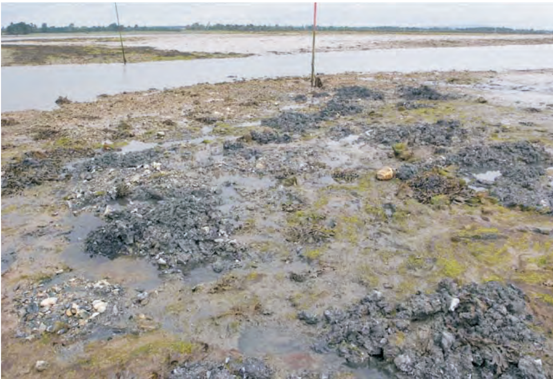
Fig 25 Damage to the Wadeway from bait digging (Maritime Archaeology Ltd 2007)
